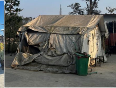
Trinagar POE (Temporary)
