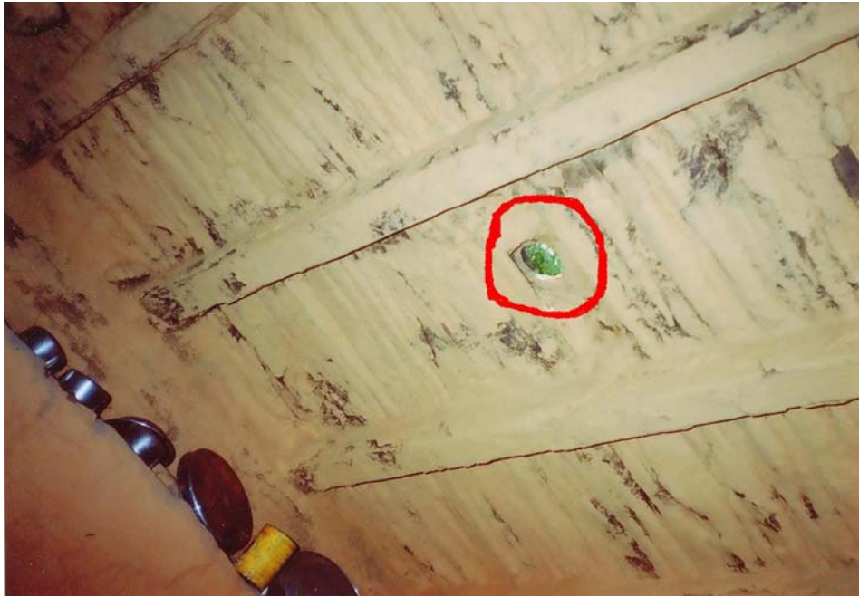
Plate 13: Hole in Roof (A type of Ventilation)
