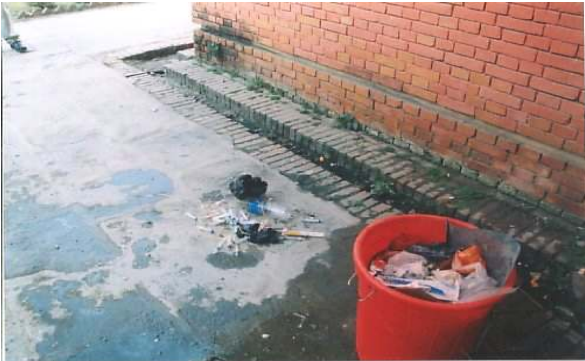
Photo 2: Dumping of used Syringe on the Floor instead of Waste Container
