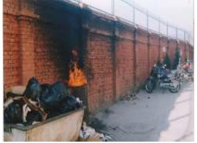
Pic 10: Store Area at Hospital with Public Reach
