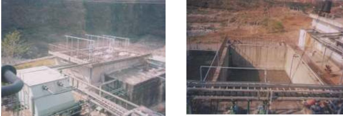
Pic 24: Effluent treatment plant at Manipal Hospital
