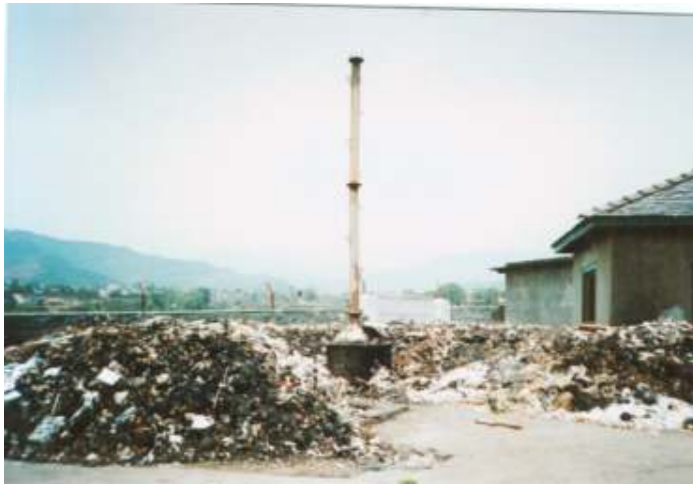
Pic 16: Open waste storage near the incinerator
