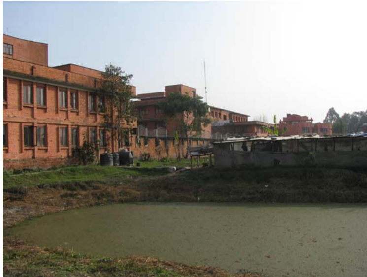
Water logged area near by Residential and Office complexes
