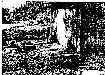
Photo 4: Poor drainage around public tap
