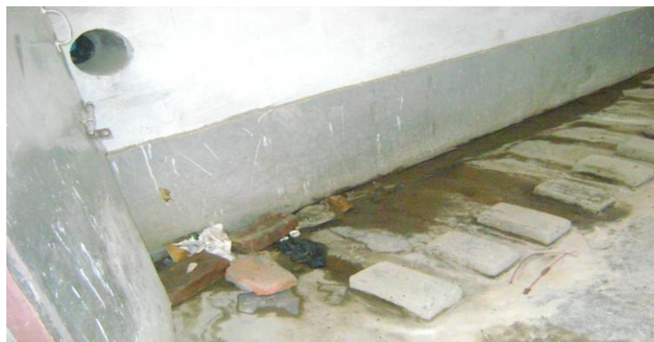
Fig 9: View of toilet with hole of pad incinerator at Butwal
